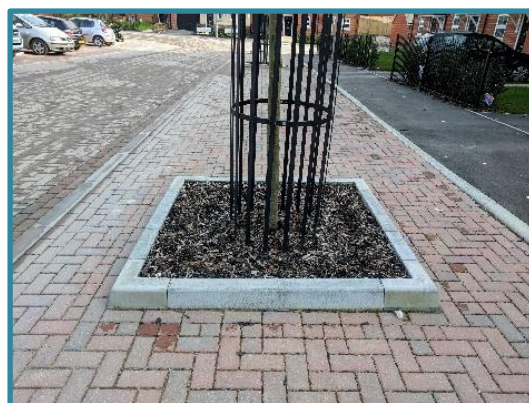
Figure 22. A well-executed tree planting within hardstanding
