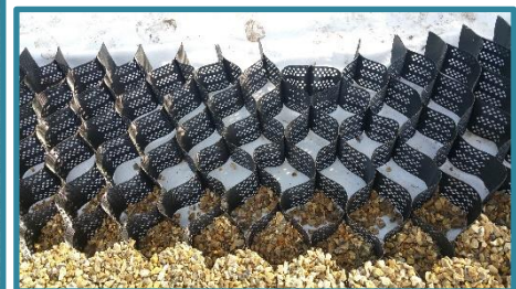
Figure 11. A cellular confinement system awaiting infill
